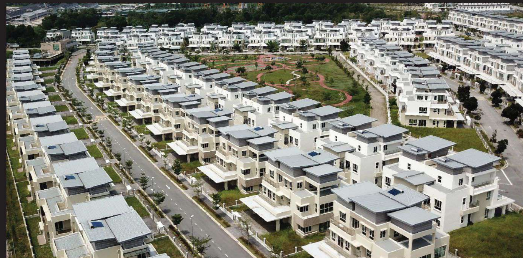
Total 49 units Solarwave supplied & installed at Regency Park housing development project at Rawang.
